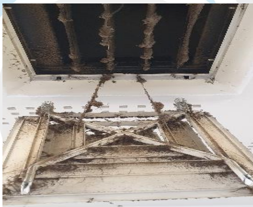
Heavy Contamination on grille and damper.
