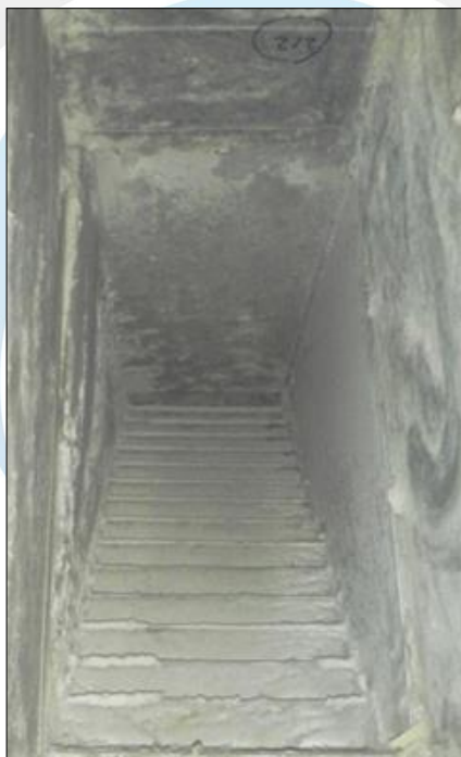
Supply duct before cleaning
