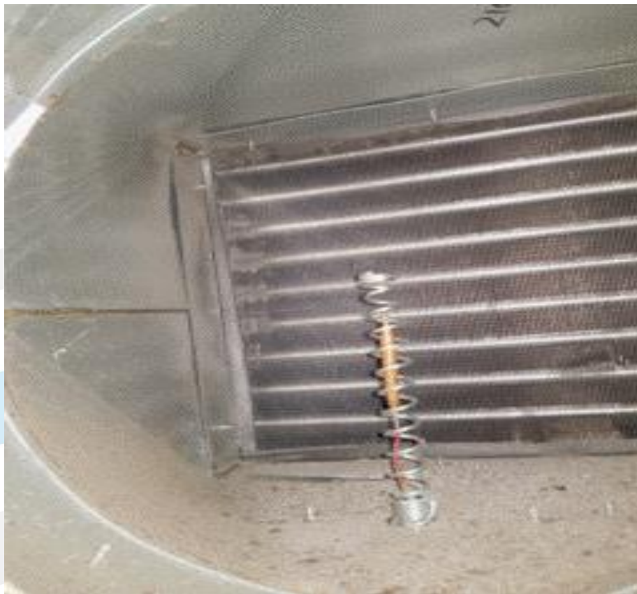
Heavily contaminated and blocked heating coil
